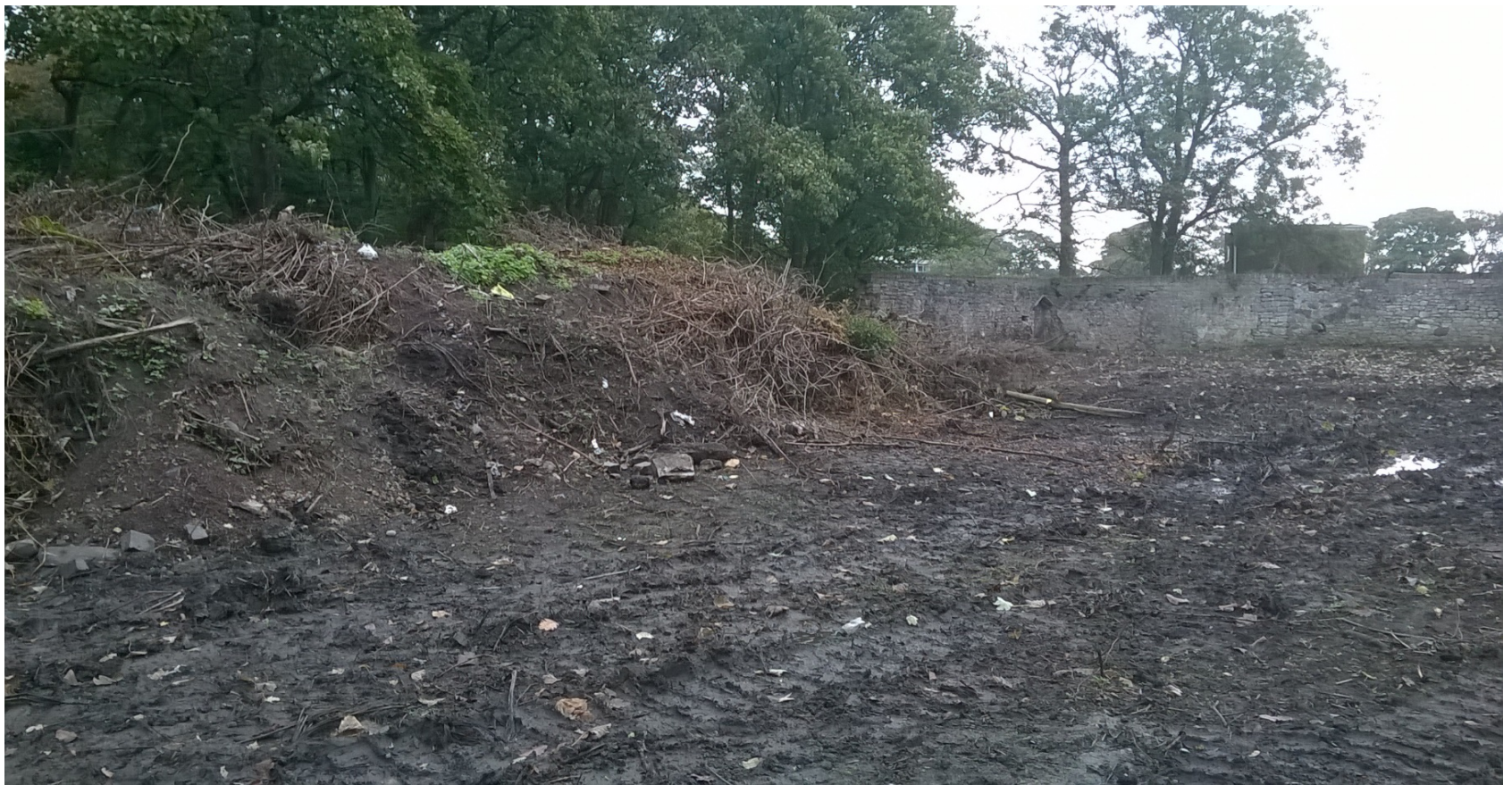
Photograph 2: View of on site stockpile
